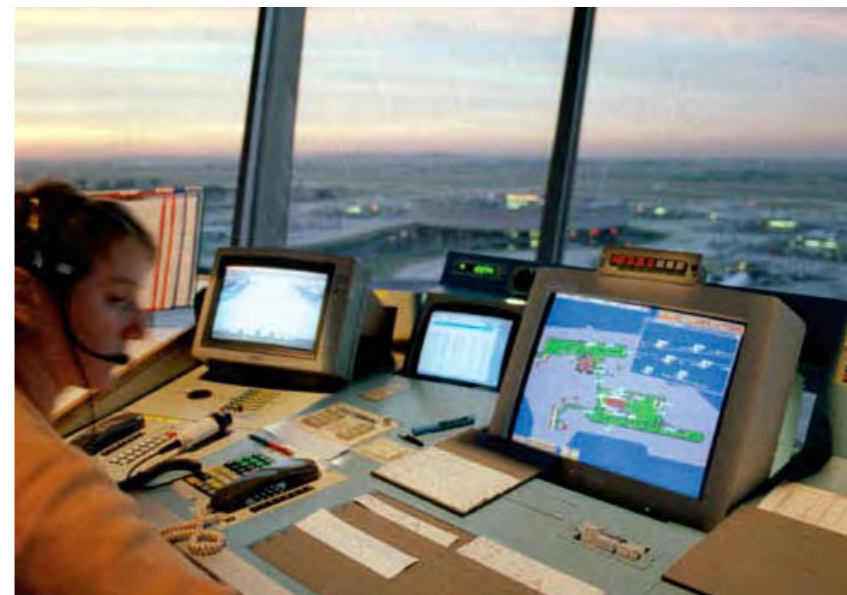
At the completion of this contract, Northrop Grumman Park Air Systems will have equipped more than 75 sites delivering communications services across half of Brazil's airspace.
