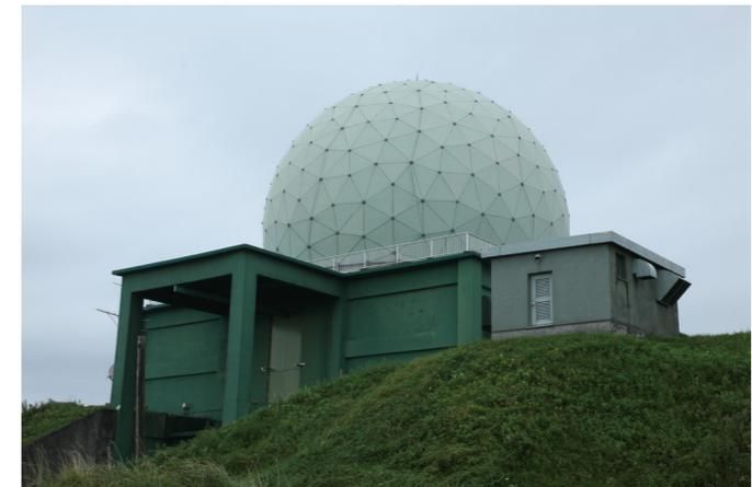
JASDF's FPS-3 (modified) air defense radar at the Tobetsu radar site in Hokkaido Prefecture. By establishing a radar on a mountain top, the radar surveillance range can be expanded. (Photo credit: Toshiharu Suzusaki)
